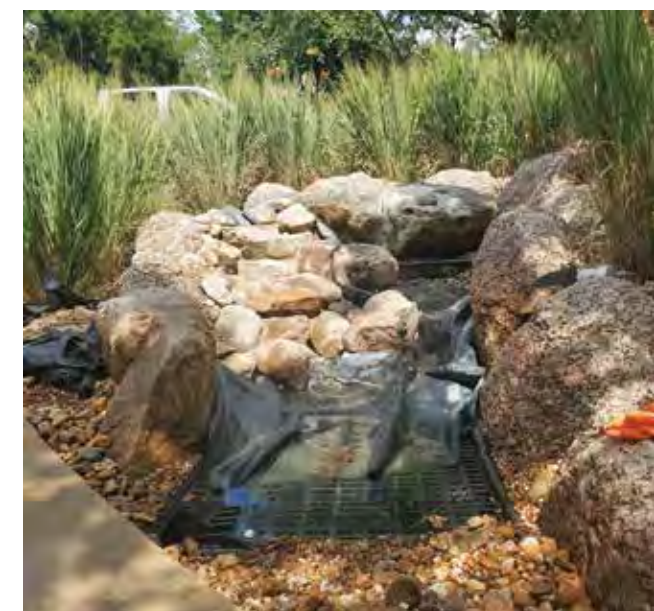
The makeover of the feature is almost complete, with most of the spillways finished. Next, we just add gravel to cover the liner and reservoir.
