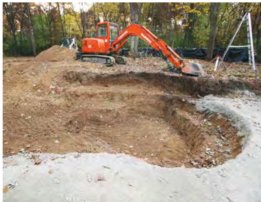
To add strength and stability to ponds, be sure to incorporate ledges (above) during excavation. Ledges provide aesthetic appeal (top, right) and create shelves for plants that require different water-depth levels. As a general rule of thumb, large equipment (bottom, right) is needed when excavating ponds larger than 600 square feet.
