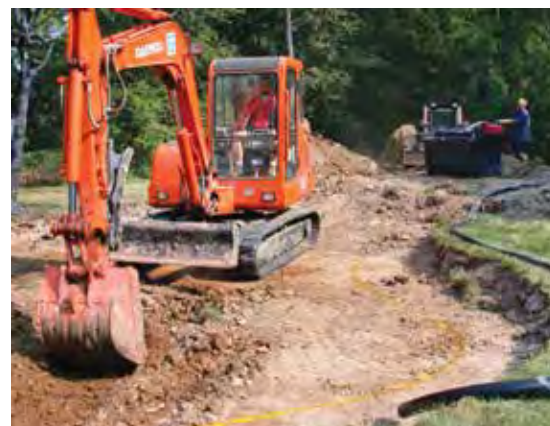
To add strength and stability to ponds, be sure to incorporate ledges (above) during excavation. Ledges provide aesthetic appeal (top, right) and create shelves for plants that require different water-depth levels. As a general rule of thumb, large equipment (bottom, right) is needed when excavating ponds larger than 600 square feet.
