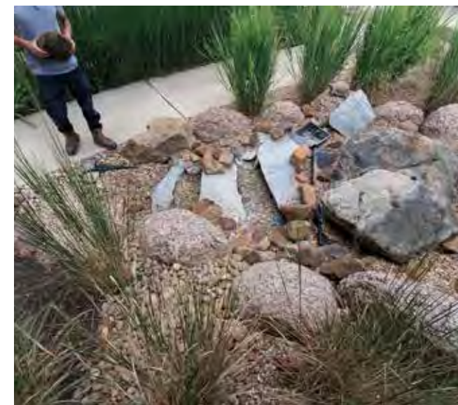
You can see an outline of the granite boulders we had to work with, along with the exposed liner peeking out from very questionable rock placements.
